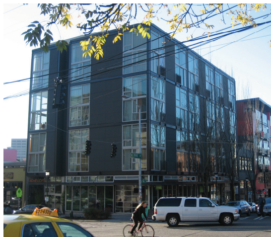
Figure 14: Successful small lot development on Pike Street.
