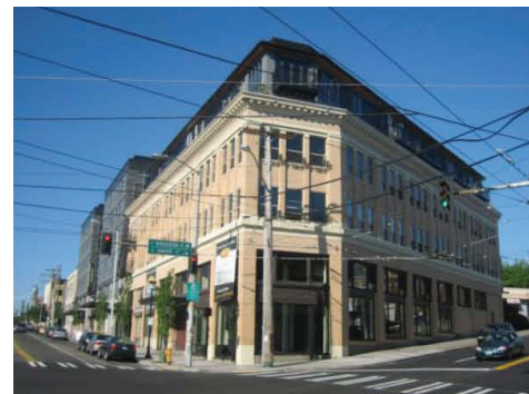
Figure 22f: Trace Lofts
