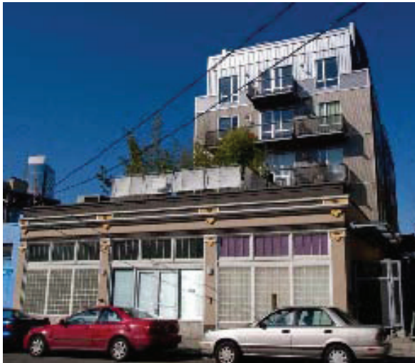
Figure 18: This addition is placed to the rear of the character structure and set well back from the street front, retaining the original proportions, scale and character of the main facade.
