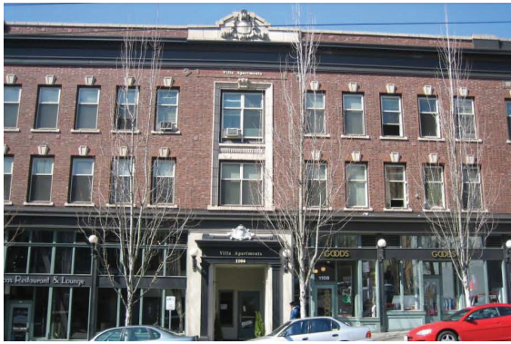
Figure 22a: Villa Apartments
