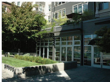
Figure 3: The courtyard of Press Condominiums provides a residential open space amenity on Belmont Avenue E.
