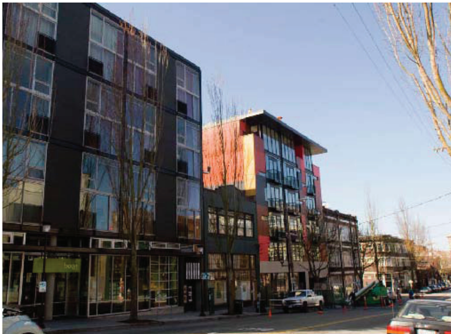
Figure B-2: Evolving streetscape maintaining compat- ible height, bulk and scale relationships.
